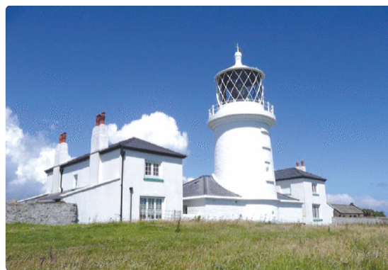
Caption: The lighthouse at Caldey Island, which is south of Wales, taken on July 3, 2008. The lighthouse is powered by acetylene gas, switched on by a sun valve. Photograph courtesy of Humphrey Bolton.
